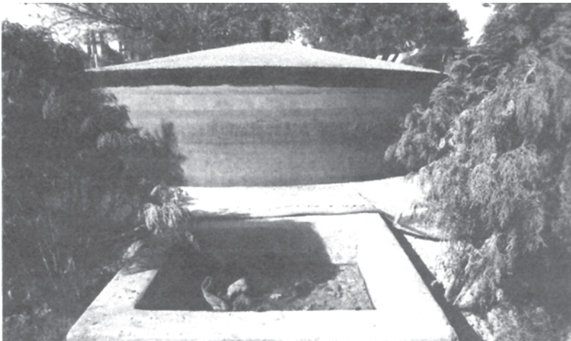
Fig.9.4 Gobar Gas Plant uses cattle dung to produce energy
