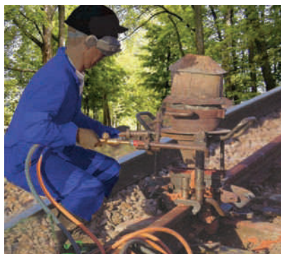
Figure 3.11 Thermit process for joining railway tracks
