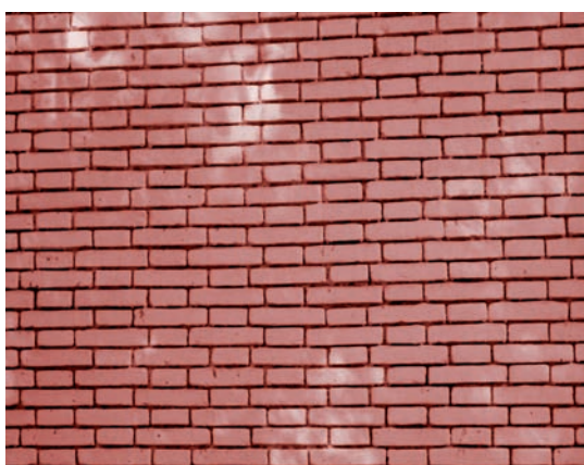
(a) Brick wall
