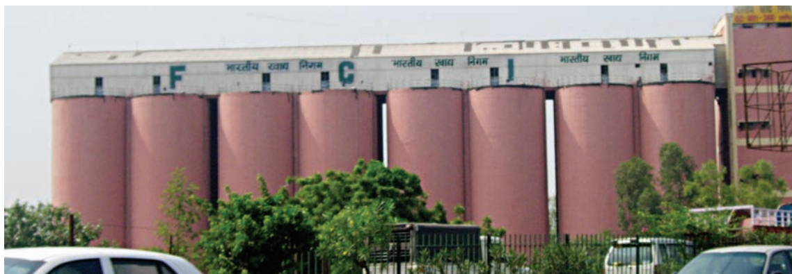
Fig. 1.10 (a) : Silos for storage of grains
